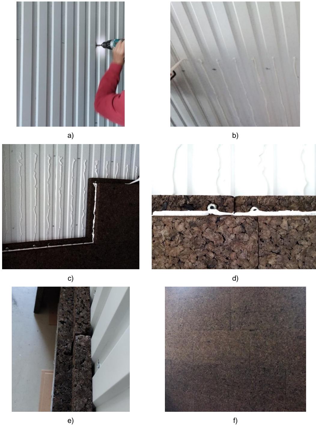
Figure B1.2: Installation of the cladding system: a) Fixation of metal sheets; b) application of adhesive sealant in rows; c) bonding of the ICB boards; d) hidden mechanical fixation and bonding through the shiplap system; e) detail of the shiplap system; f) final aspect of MD FACADE cladding system.
